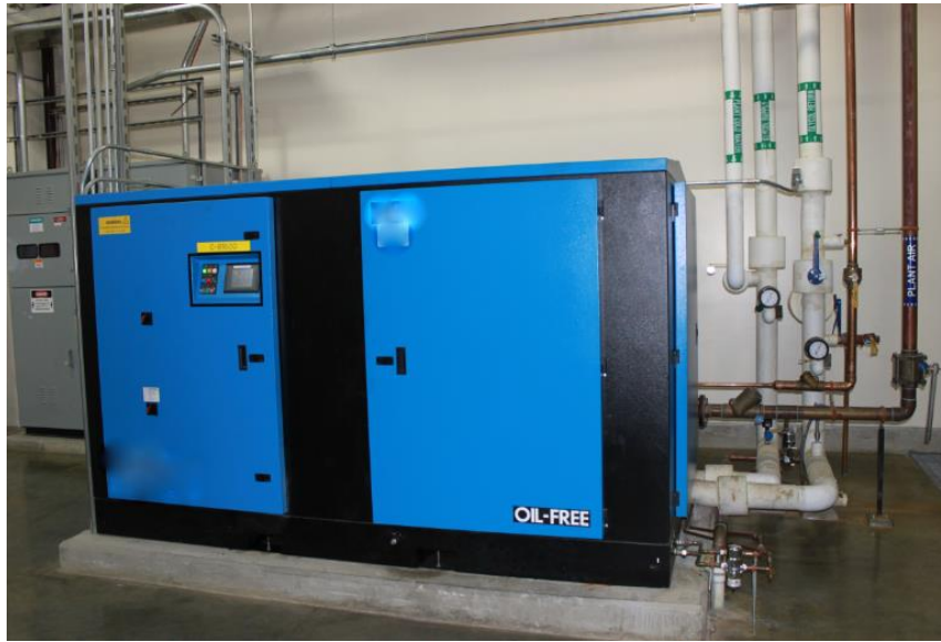
Figure 2-4. Plant air system, which can help maintain air quality and humidity standards in a facility
