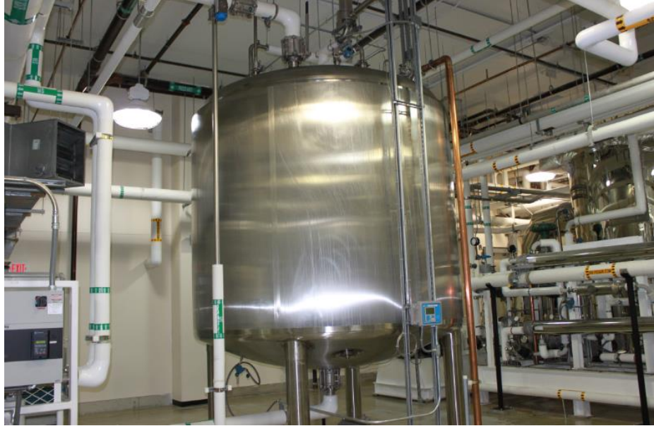
Figure 2-14. Tank holding Water For Injection (WFI)
